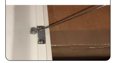
**2.** Fix the ceiling brackets into place, using the long screws and wall plugs provided.
